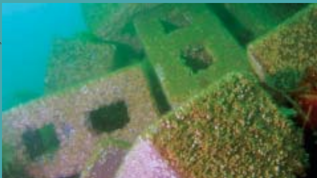
Complex blocks (each measuring 40cm x 20cm x 20cm) of the Loch Linnhe Artificial Reef shortly after deployment.
